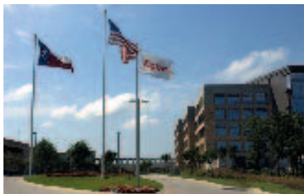
Sabre's Southlake building, home to some of Sabre's 7,000 employees.
